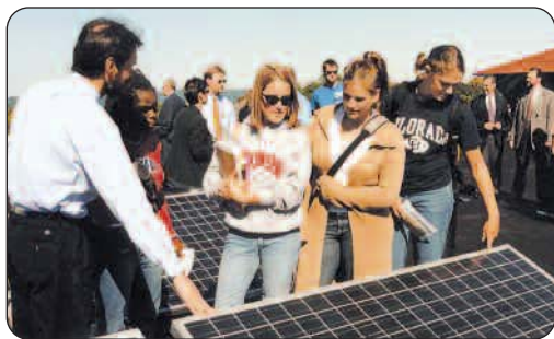
The Madison Gas and Electric Foundation donated 10 Photovoltaic systems to area high schools. The units produce electricity for the schools while serving as a learning tool for several curriculum areas.
