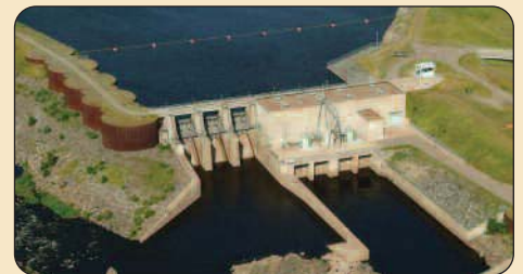
Xcel Energy’s Jim Falls hydroelectric power plant in Chippewa County.
