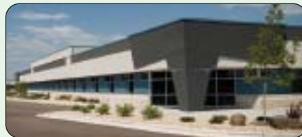
Suttle-Straus' East Building by the Renschler Company
